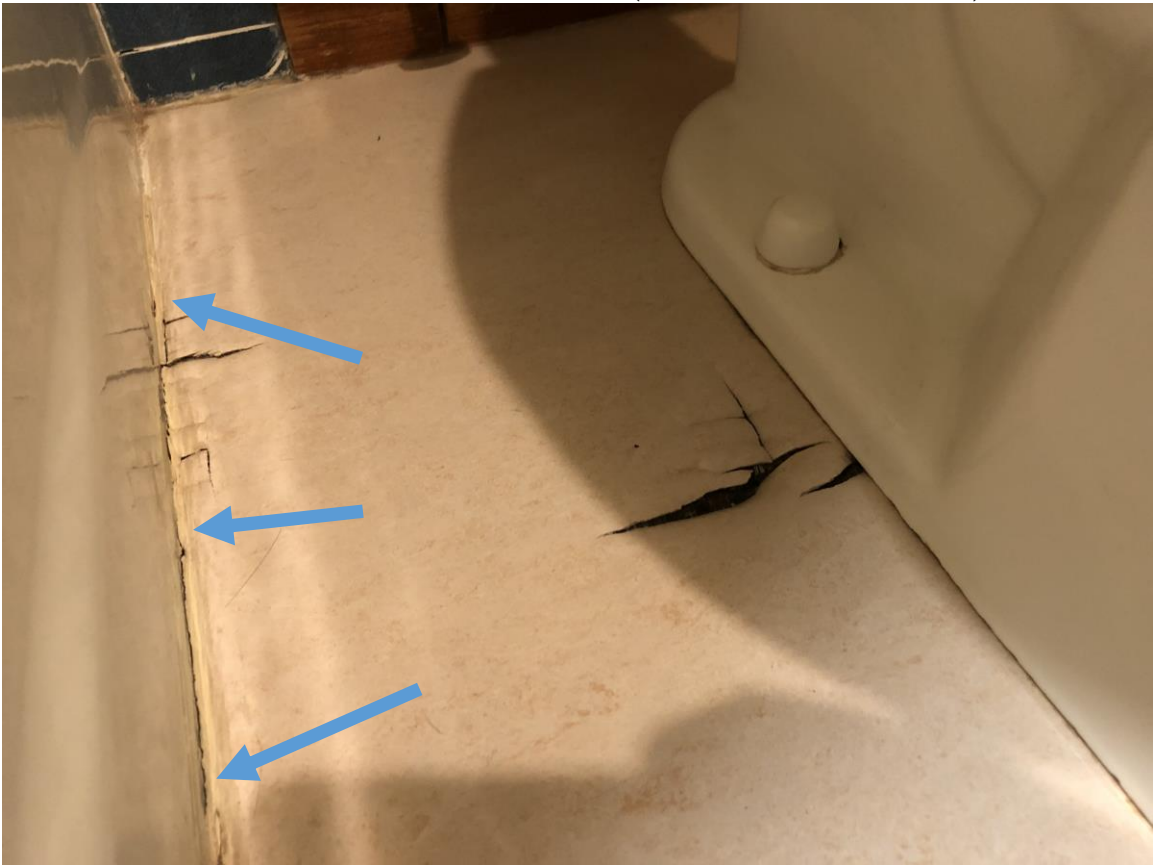
Room 310 toilet base has a leak (see arrows above).
