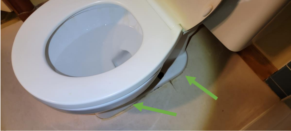
Room 310 toilet base has a leak (see arrows above).
