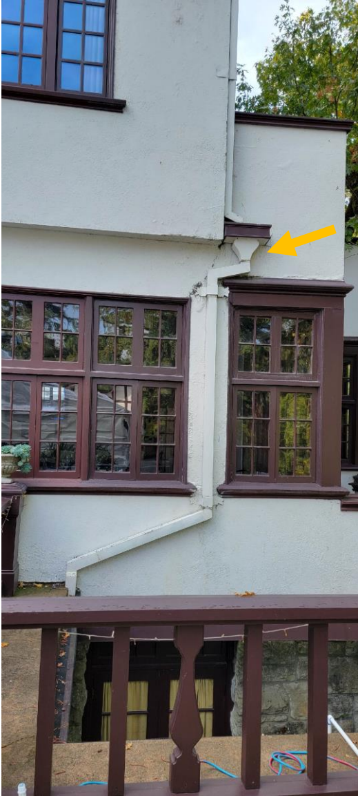
Dining outside wall
